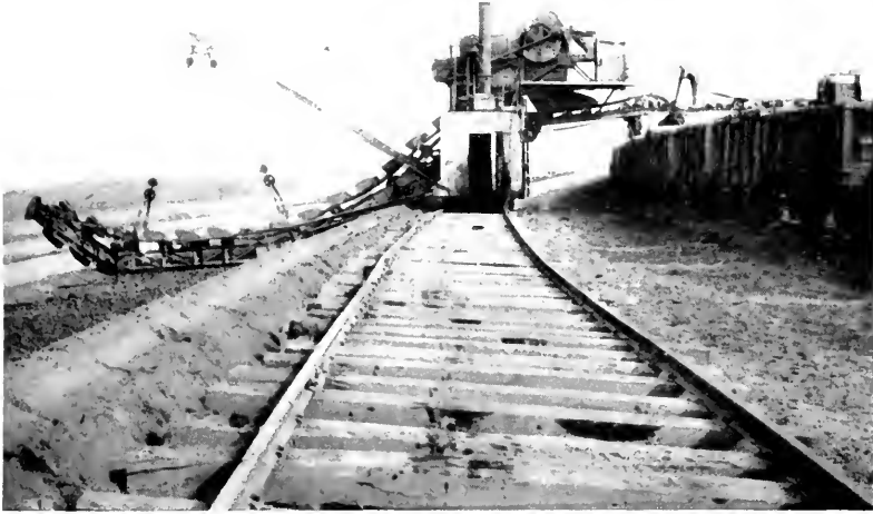
THE EXCAVATOR AT WORK, DIGGING A CHANNEL FOR DRAINAGE (OCT. 7)
