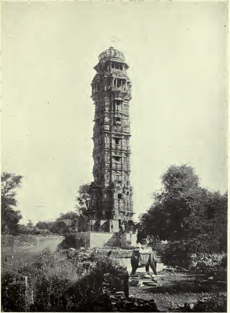
JAI STAMBHA AT CHITORGARH (A.D. 1451): THE TOWER OF VICTORY
