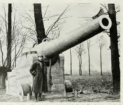
A big gun that will never fire a shot. A genius in the French army conceived the idea of building a dummy gun out of papers sent to the soldiers at the front, and the result is shown in the photograph. It looks like a 240 millimetre gun, and concealed in a wood, will be spotted by enemy aviators and will draw many shells from their big guns. But no one will be hurt
