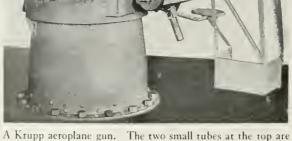
Krupp aeroplane gun. The two small tubes at the top are filled with glycerine to take up the recoil
