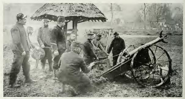
A French device for breaking through wire entanglements
