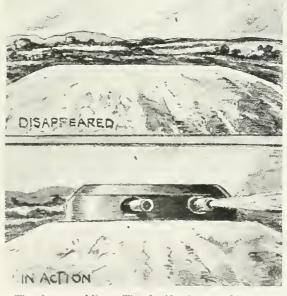
The forts at Liège. The fortifications at Liège were planned by the Belgian engineer General Brialmont. One of their most effective features was the disappearing turrcts, in which the guns were mounted
