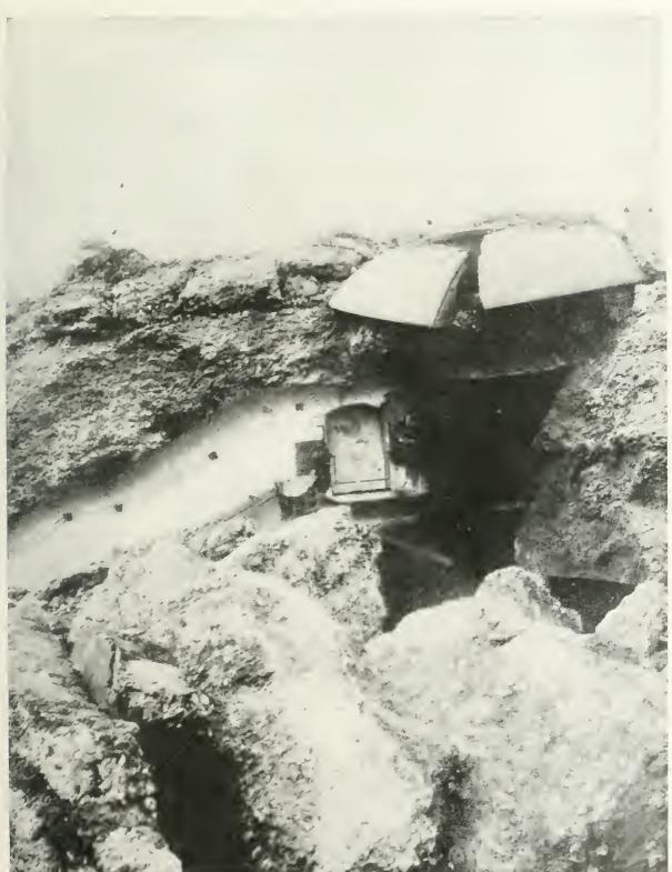
A RUINED LIÉGE FORT A steel turret overthrown and masonry demolished by German siege guns
