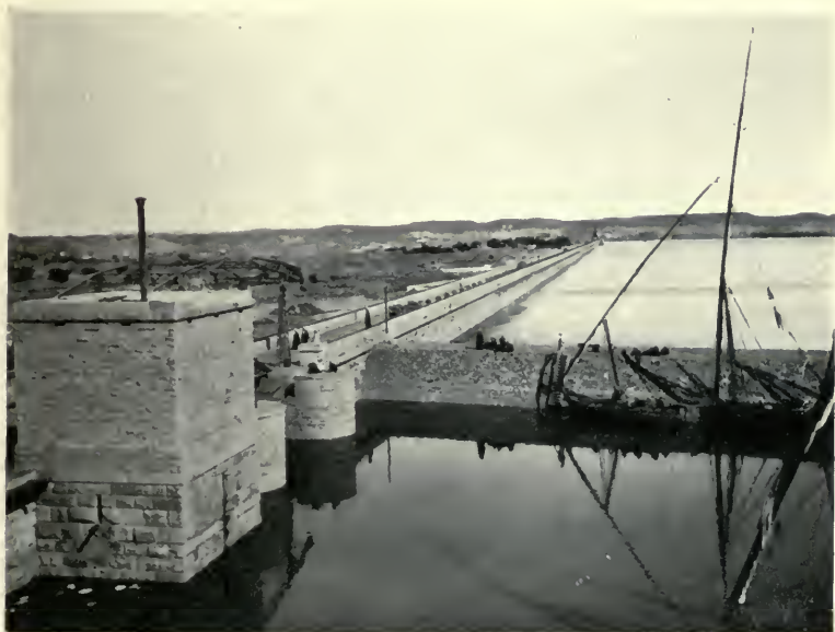
LOCK, BARRAGE AT ASSOUAN
