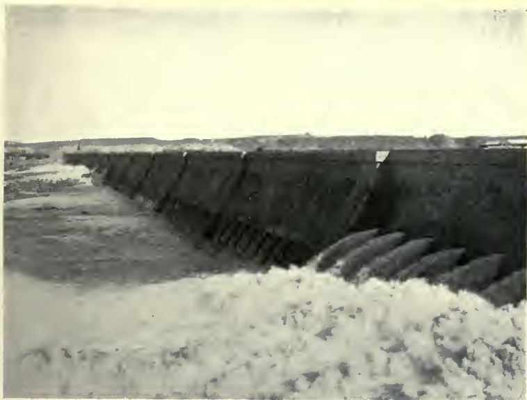
THE BARRAGE AT ASSOUAN
